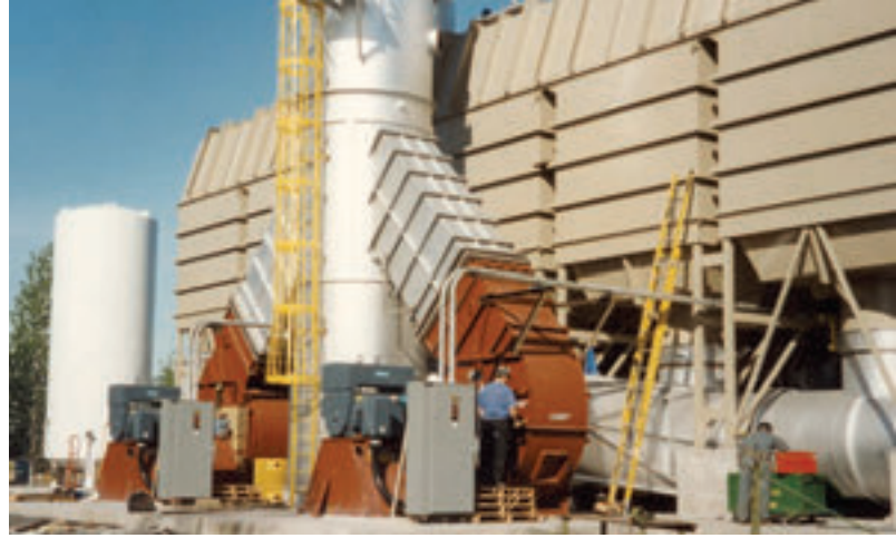
Two Series 4000 BCI fans (500 hp, 1800 rpm, 60" diameter) installed on a regenerative thermal oxidizer.
