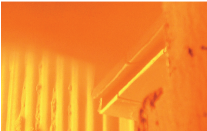
With a combination of measures including staged combustion, fuel / air mixing and firing through new Ultra-Low Nox burners, RJM achieved a NOx reduction of greater than 50% at this T-fired 440MW coal / oil power station.
