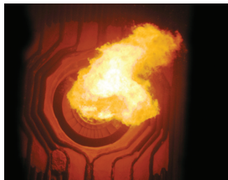
An RJM Ultra-Low NOx oil burner under full load.
