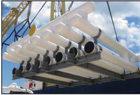
Slug Catcher (Modularized for Shipping)
